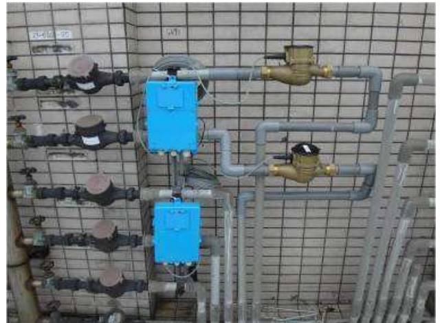
Graph 3. On-site electronic water meter installation condition
